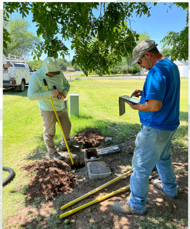
Fig. 1: Staff digging up and visually inspecting water lines for material verification and classification.
